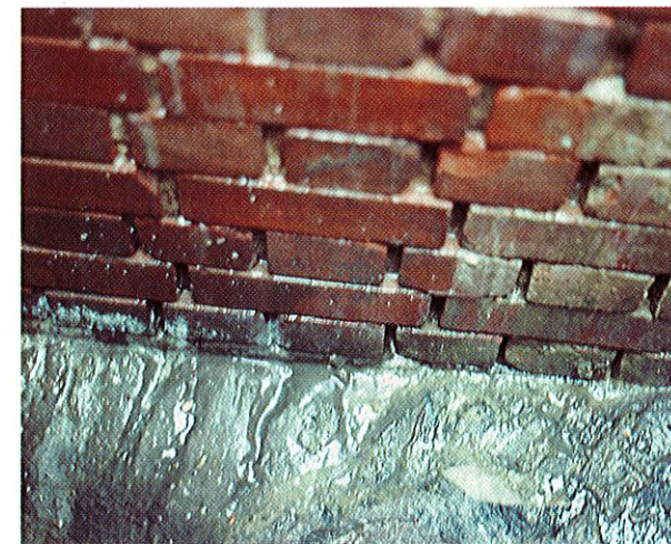
Attack by sulphuric acid oxidised from atmospheric hydrogen sulphide in the presence of moisture at a pressure main outfall. Most of the mortar between the clay bricks has disappeared and the concrete benching has been severely attacked.
