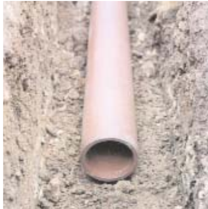
Clay drainage with trenchbottom bedding
