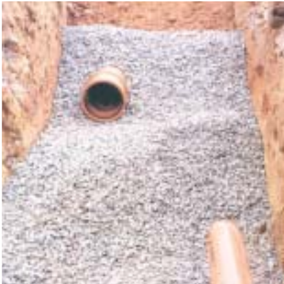
Plastic Drainage with full surround
